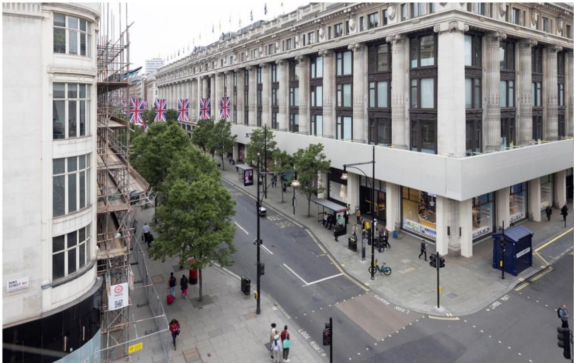
Current view towards the west – Duke Street junction
